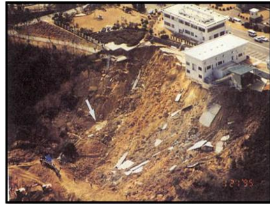
Fig. 16: Landslide during Kobe earthquake (1995)
