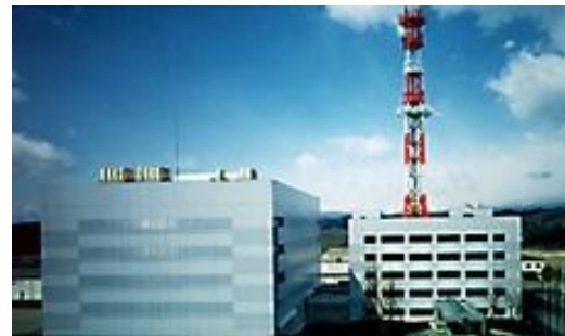
Base Isolation at Computer Center for Tohoku Electric Power Company in Sendai, Miyako prefecture, Japan
