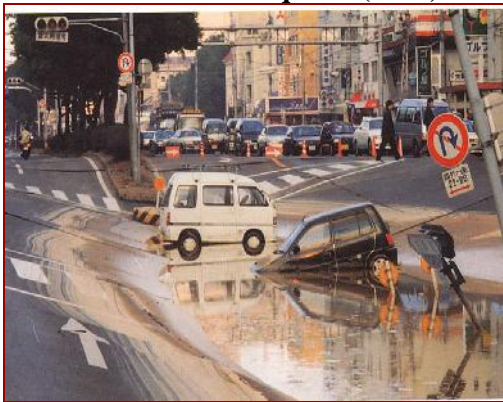
Fig. 17 : Liquefaction failure in Kobe leading to subsidence & ground water coming up (1995)
